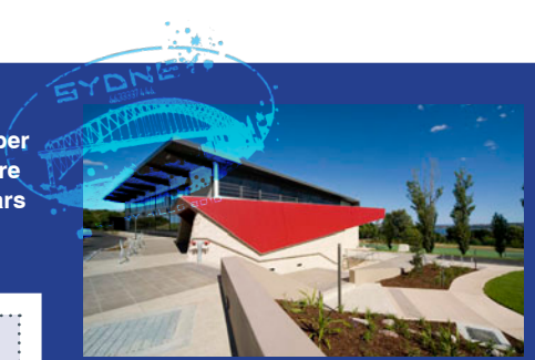
The Marie Bashir Mosman Sports Centre completed by MODE DESIGN in December 2010.
