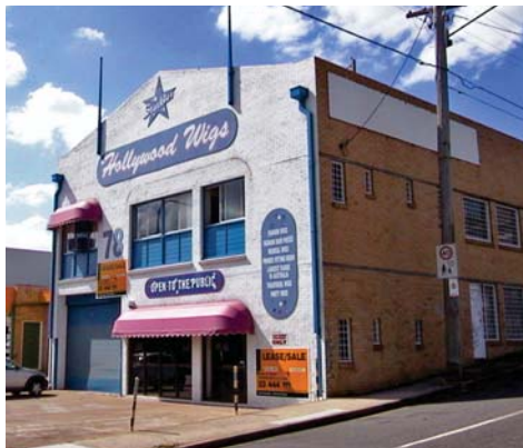
Brisbane studio building prior to its internal and external refurbishment
